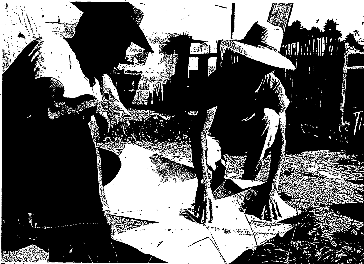
Training home construction crew, Guatemala.
