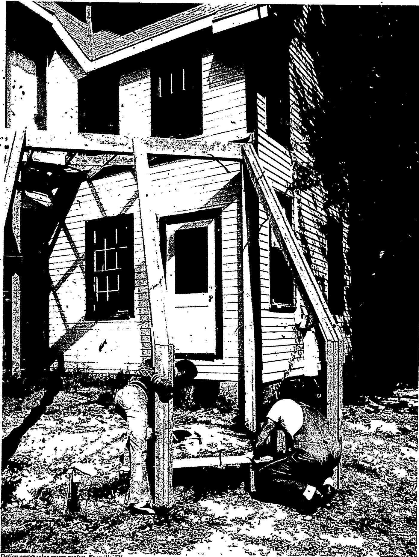
Design center solar energy project, Knoxville, TN
