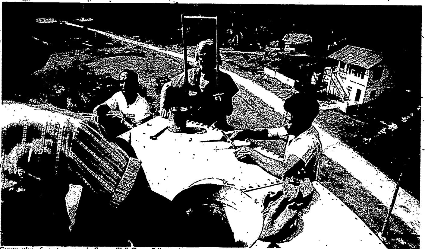
Construction of a water system in Orange Walk Town, Belize.
