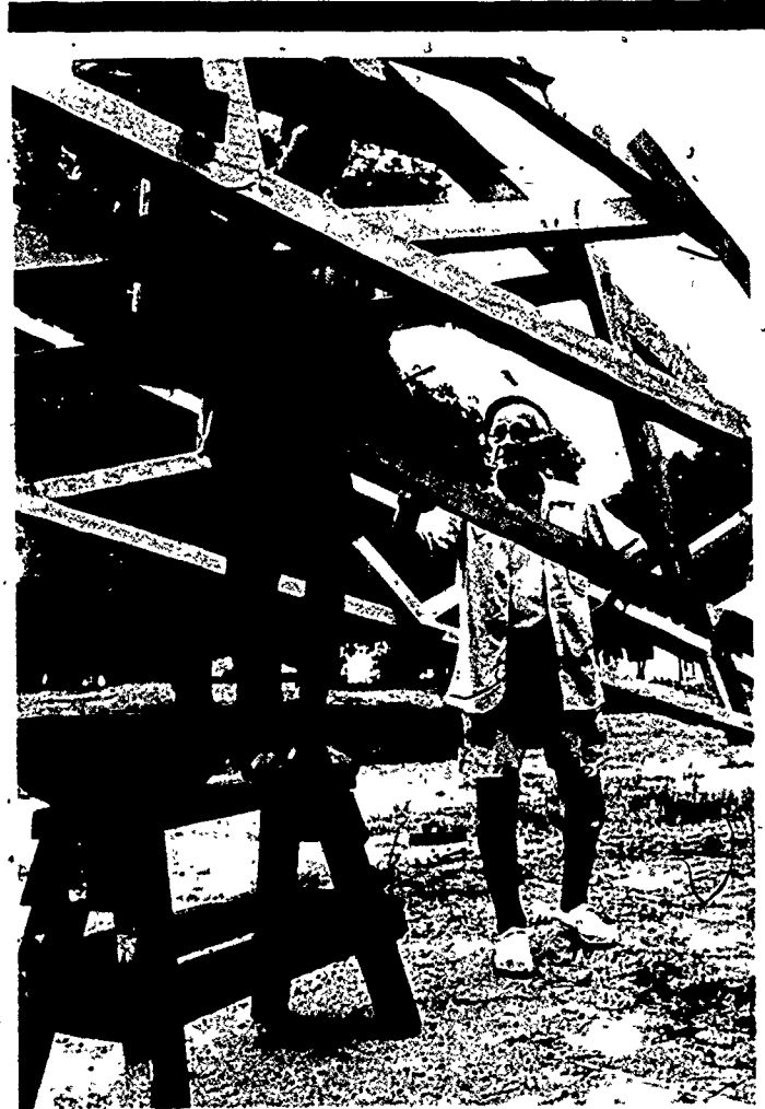
Peace Corps volunteer and workmen working on roof trusses at Bunumba Teachers College, Sierra Leone.
